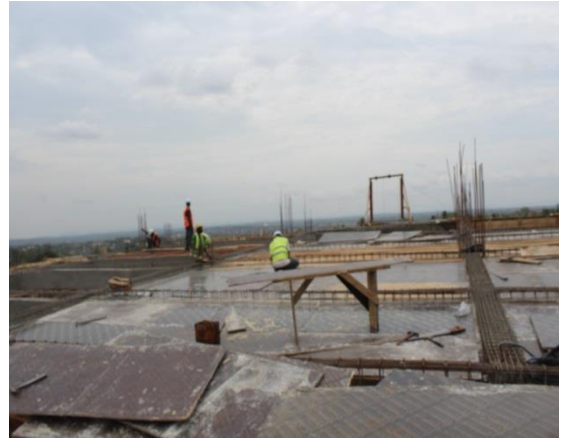
Coffrage dalle R+2
