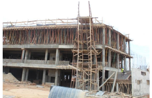
Coffrage dalle R+2
